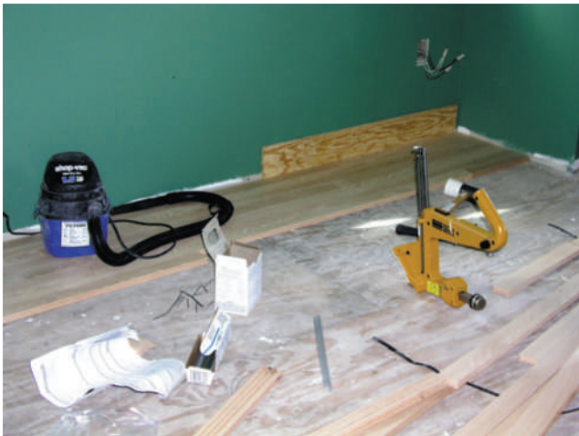
FIGURE 1-9 Carpenters install hardwood floors.
