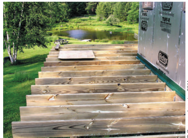
FIGURE 1-6 Joists set for a deck by carpenters.
