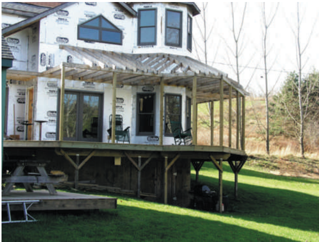
FIGURE 1-8 Porch roof framed by carpenters.
